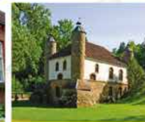
Heimtal Manor Complex
